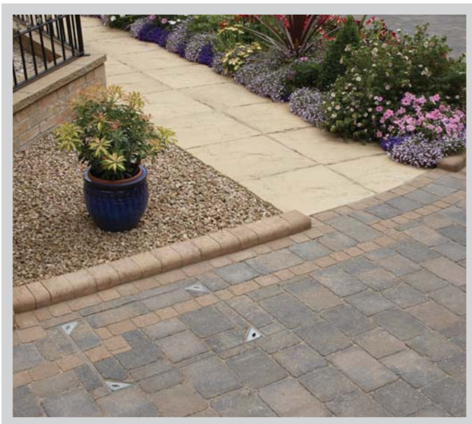
Blocks mortared into position around a cover
